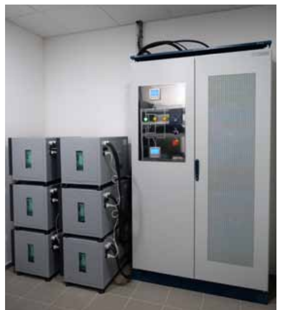
Example of the use of hybrid photovoltaics in Zlín: energy from solar panels is stored in 6 batteries with a total capacity of 51 kWh
