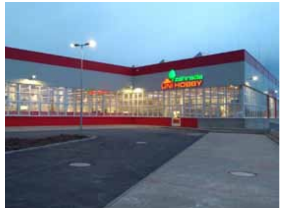
For Uni Hobby Svitavy, we carried out electrical installations for a total of 37 mil. CZK
